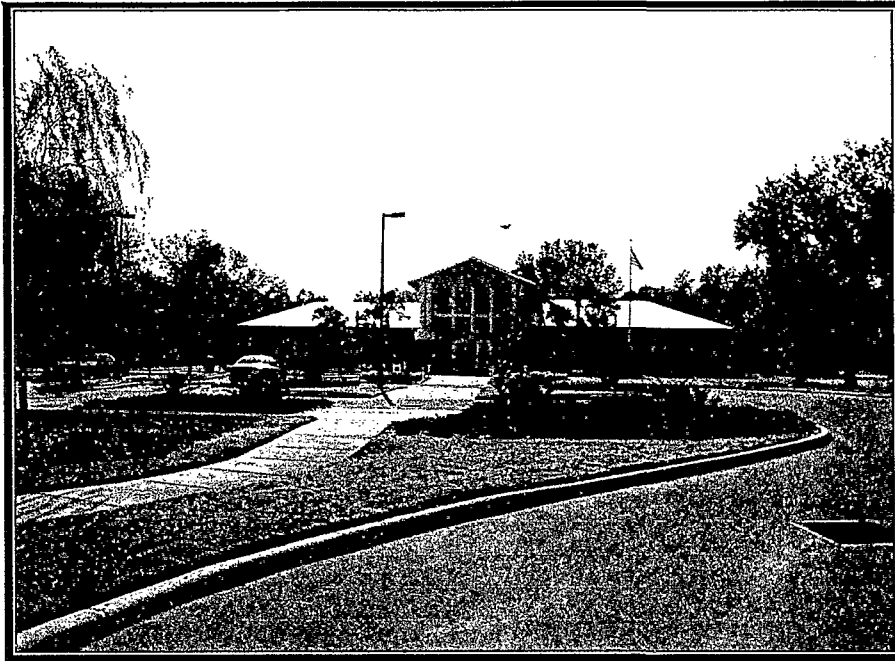
Photograph 7: View to the south of the Moore Center
